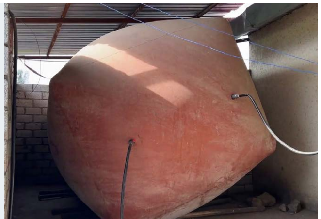
Energy Bio digester at Zagol milk, AINFP Client in Ethiopia. Photo: AINFP
